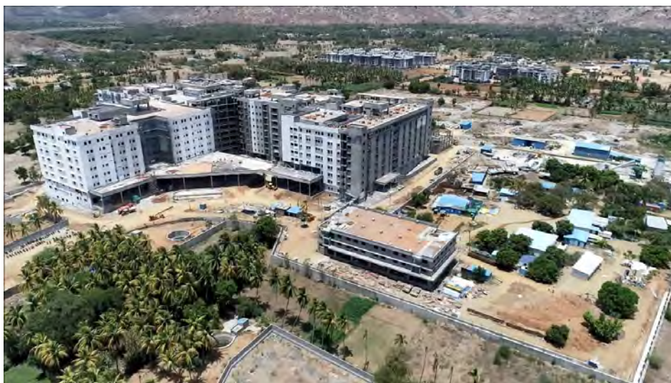
CMC Kannigapuram Campus, now nearing completion.
